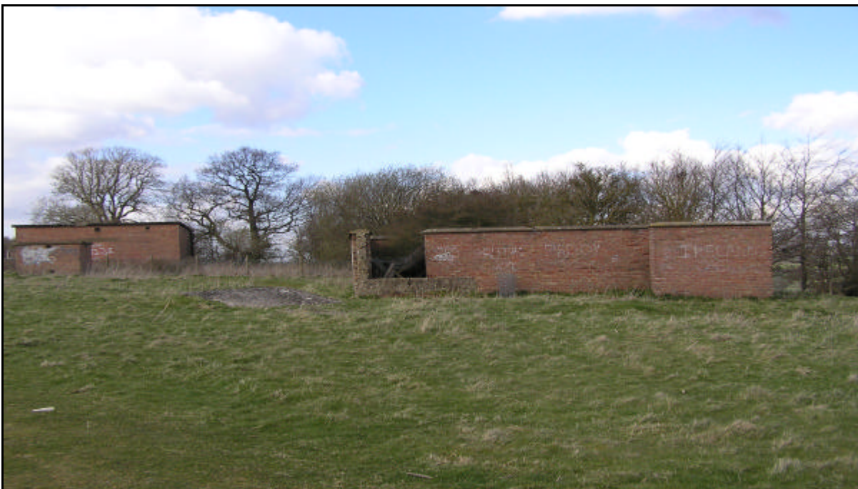
Blast pen on the right of the picture. Note concrete block on ground immediately to its left
