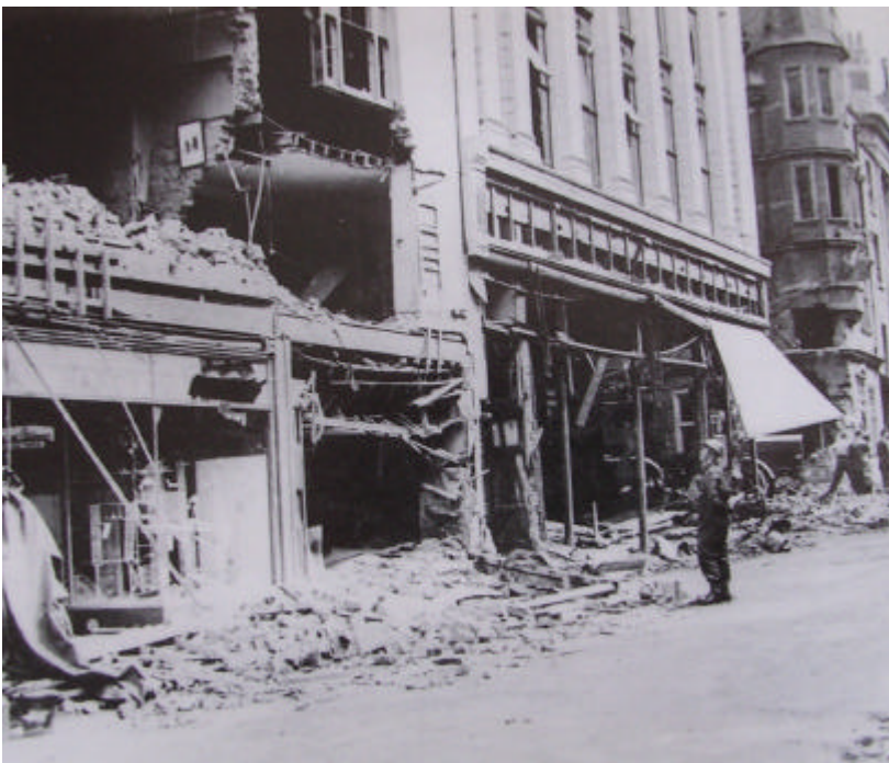
Damage to the shops in Gold Street
