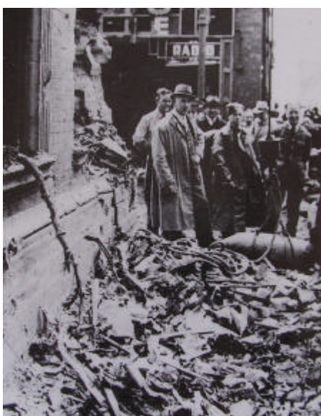
Debris and damage to shops in Gold Street
